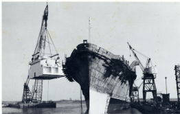
The Sun 400 lifts the bow up to the deck of a vessel under construction.
