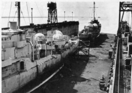
Filling the dry docks and berths to capacity, the task of Ship Repair Sales, is best reflected in this photo of two destroyers simultaneously dry docked on No. 3. By rearranging the blocking, four destroyers at a time can be handled.
