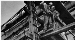
Stage Builders such as these two employees work at great heights to erect the staging which will be used later by other members of the shipyard in their work.
