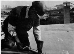
Gouging a butt weld is one of the duties of the chippers.
