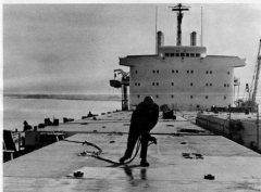
A member of the Paint Shop sprays the deck of a ship during a construction stage.
