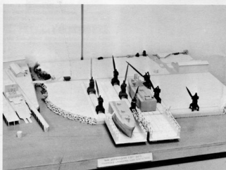
MODEL OF SUN SHIP'S PROPOSED NEW FACILITIES BUILDING PROGRAM SHOWS SEPARATED DRYDOCK SECTIONS being used independently to move half ship sections from building slab to water.
