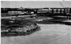
On the left, progress on the landfill is shown (about 20,000 cubic yards of clean fill had been dumped when this picture was taken).
