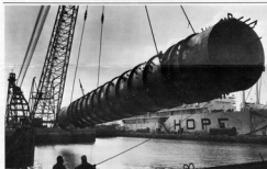
SUN "800" PLACES 320-TON CRUDE OIL TANKER on board vessel for shipment to Hong Kong's refinery in St. Cruz, U.S. Virgin Islands. The crude oil tanker is 200 feet long with an inside diameter of 19 feet and has a 5/8 inch average wall thickness that includes a dual stainless steel liner. The tanker left Sun Ship on Tuesday, February 19th, aboard West India Line's INAGUA LIGHT which docked here to make the pick-up.
