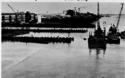
At the right, pile driving on cell 16 is taking place. The cell is a steel structure that will act as a bulkhead. The cells are in front of the old pier—a total of 31 of them will form a 1200 foot pier at completion.
