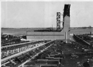
THE FIRST SECTION OF SUN SHIP'S NEW FLOATING DRY DOCK slides down the launching way. The dry dock section is 350 feet long, 114-1/2 feet wide and weighs 3,300 tons. When completed, the dry dock will be composed of two 350 foot sections that, when used together, will be capable of lifting up to 70,000 tons. The shipyard's present dry dock is capable of lifting up to 44,000 tons.
