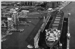
Photographed in Sun Ship's new #4 dry dock is the 40,967 gross tonnage carrier "Helga Oldendorf" of Singapore registry. The vessel is owned by Hagen Oldendorf of Lubeck, Germany. The photograph shows the progress of improvements accomplished in the yard to date.
