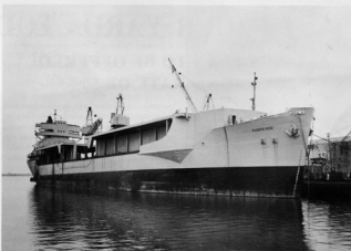
The Puerto Rico, a U.S. Navy vessel, is moored in Sun's #4 wet basin while it undergoes repairs including underwater plate renewal as well as internal offhull repair and replacement. The 560-ft. vessel is a T-2 tanker built in 1944 and jumboiled in 1967. The Puerto Rico's most recent service
