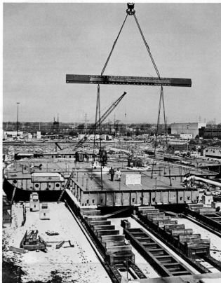
The keel for the JOHN B. WATERMAN is placed on "A" slab in the North Yard. The placement of the 118-ton center line double bottom marks the start of
