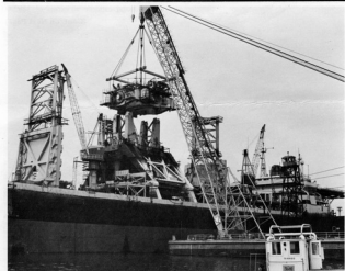
The SUN 800 places the gimbal on the Hughes Glomar Explorer. The lift, amounting to 630 tons, was the heaviest in the entire construction process of
