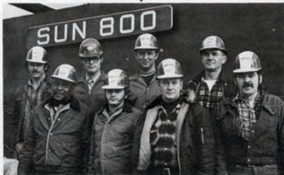
A new era began October, 1972, at Sun Ship when the Derrick Barge Crane—Sun 800—came to life. This equipment has made possible the construction of Hughes Glomar Explorer and will lend itself to many other unique shipbuilding possibilities in the future. With pride, Management salutes the men of the "800". They set an example of the team work needed at Sun Ship to continue
