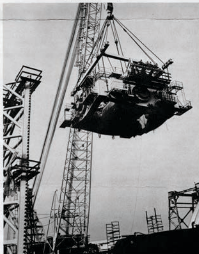
Through the efforts of the men shown above, probably the heaviest single lift on the East Coast took place here at Sun Ship when the Sun-800 hoisted an inner and outer Gimbal platform of around 735 tons aboard the HUGHES GLOMAR EXPLORER. Estimated worth alone of each bearing is 1/2 million dollars; there are four bearings on this platform.
