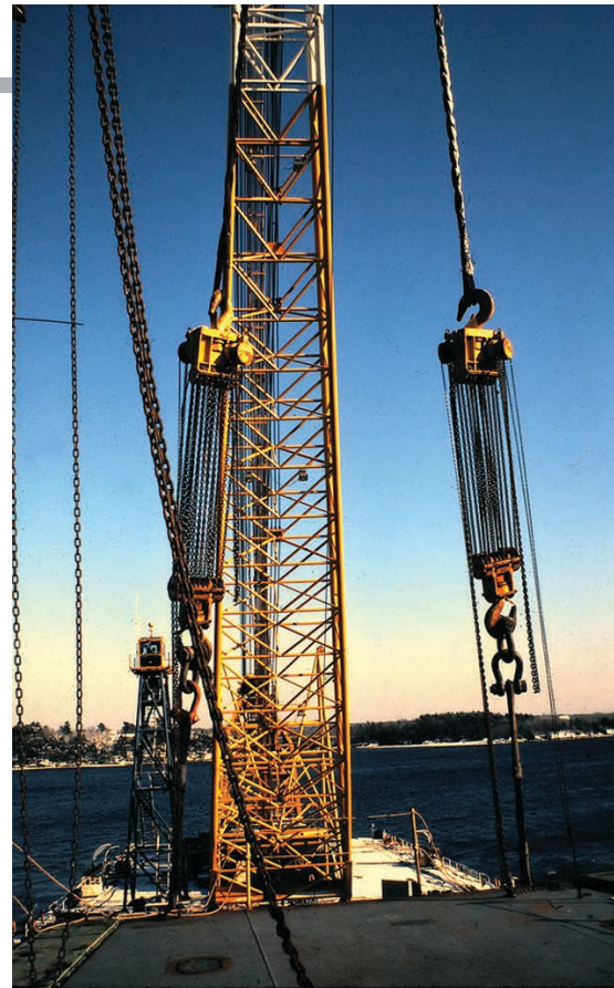
The SUN 800 places the last unit for the Sugar Barge that was being built for Sun at Bath Iron Works in Maine. Photo courtesy of Rich Janney
