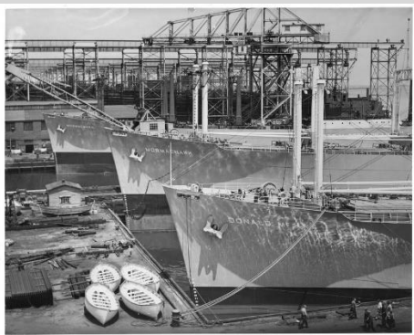
5.4: Photo taken of Sun Ship's CY 'Outfitting Basin' showing L/R: 'MORMACWREN' H-177 at 1-Pier, 'MORMACHAWK' H-176 at 2-Pier South and 'DONALD M c KAY' H-175 at 3-Pier North Photo ID: 74319247r7
