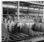
The deck subassembly was constructed upside down and includes the longitudinal and transverse bulkheads. Ten such subassemblies were constructed; the deck subassembly was then turned over and placed on the already constructed bottom shell assembly.
