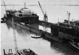
Midbody section being parted from stern section.
