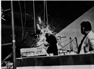
MRS. EDWARD LaCROSS shown christening the barge, which will house the crane, at Kelo Marine Inc.'s Galveston Yard, June 23, 5:30 PM. (Both photos compliments of E. LaCross, Hull Superintendent)
